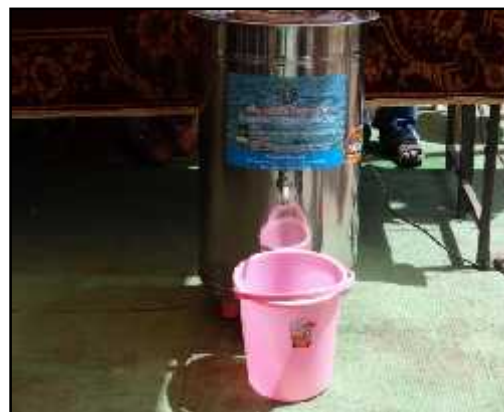
Chemo- Defluoridation Units installed in Sakhara and Chichkavatha villages
