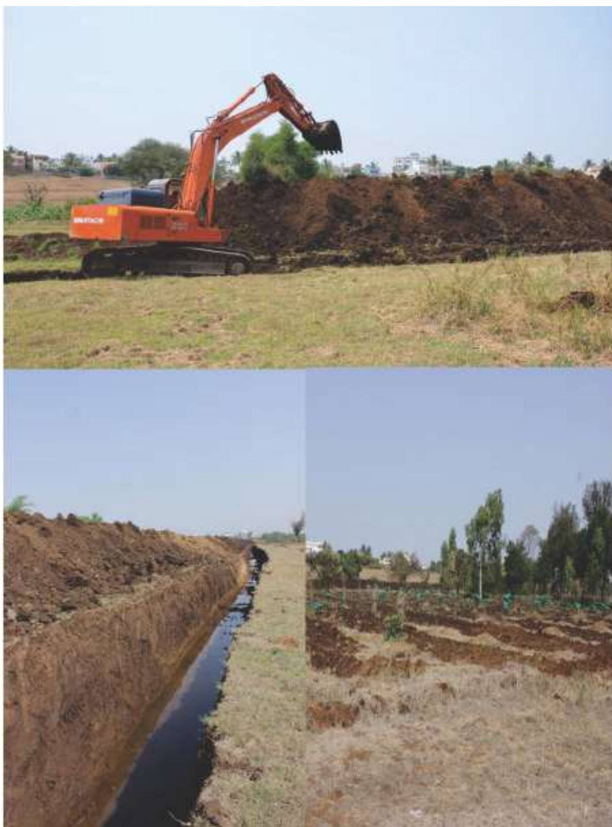
Plate : XXXX: Trench and Land preparation
